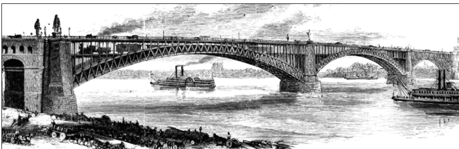
Figure 2: The St. Louis Bridge built by James Eads (Williams 1877)
