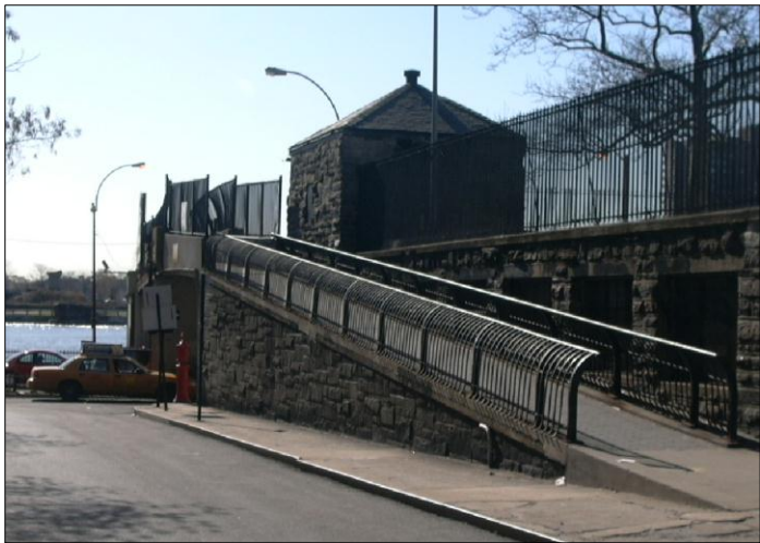
Figure 6. West ramp along 78 th Street.
