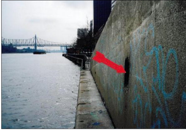
Figure 4. The East River bulkhead line looking south. The Queensboro Bridge is in the background and the wall supports the ramp.
