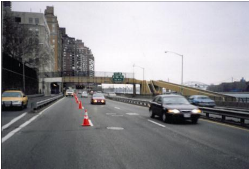
Figure 2. The bridge elevation looking north. Note the stairs and the ramp along the East River esplanade.
