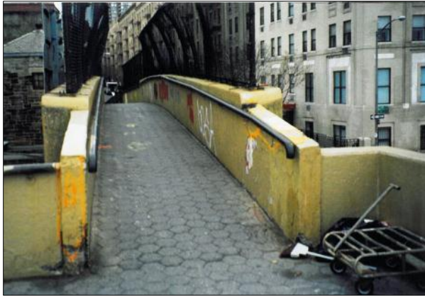
Figure 5. The pedestrian bridge looking west.
