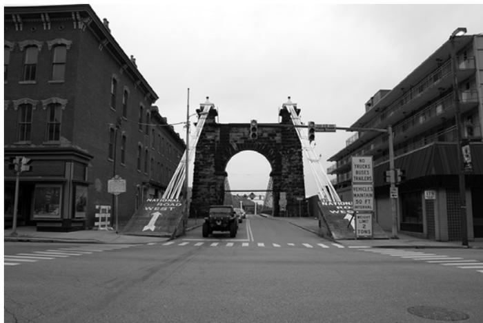
Figure 6. Tower and anchorages Wheeling Bridge (Gralian 2014)
