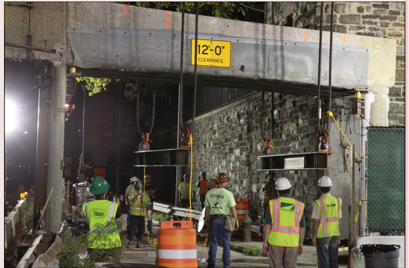
Preparing to remove the side span of the bridge.
