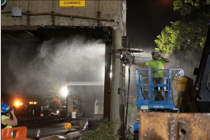
Cutting the pier and preparing to remove the main span.
