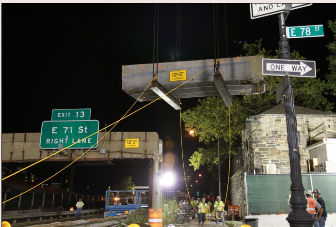
Removing the side span of the bridge.
